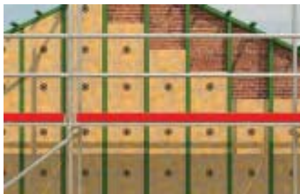
Insulating materials in rear-ventilated façades
