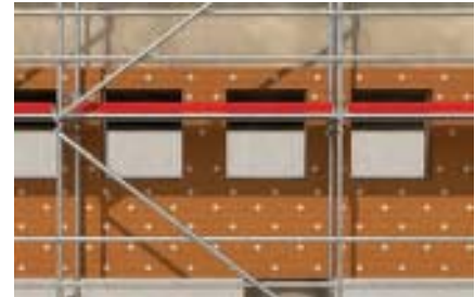
Pressure-resistant insulating materials in curtain façades
