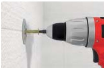
Screwed fixing of insulation boards
