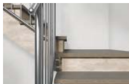
Stair treads on concrete stair stringers
